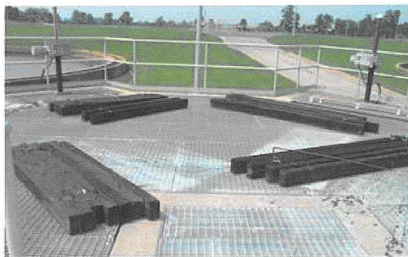
Distribution box - Top view
